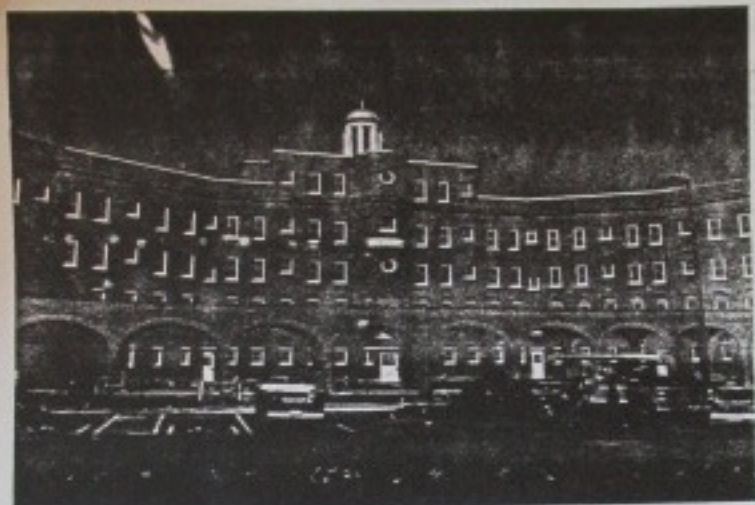
REAR VIEW OF ROBERT MILLS BUILDING AND COLONNADE
