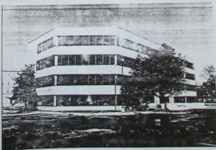
VIEW OF NEW BUILDING FROM SOUTH WEST
