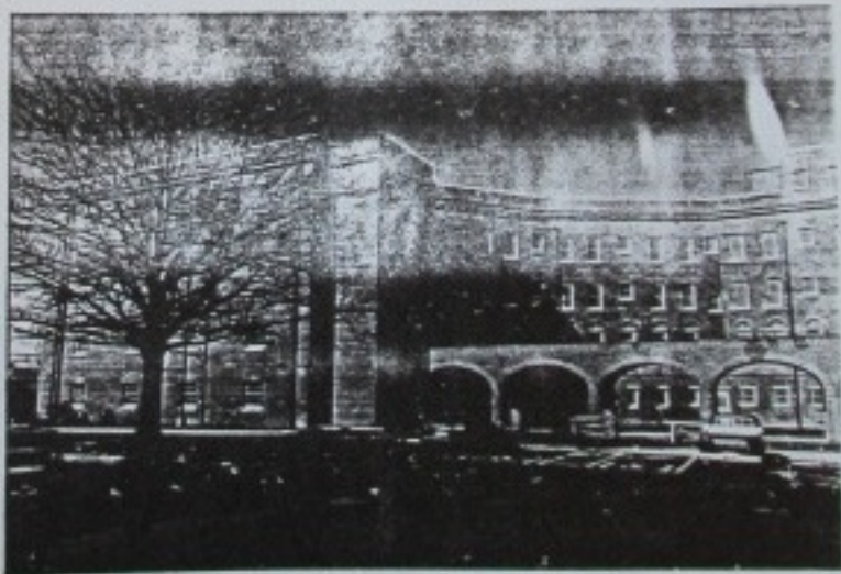
WEST WING, NEW COLONNADE AND ELEVATOR TOWER
