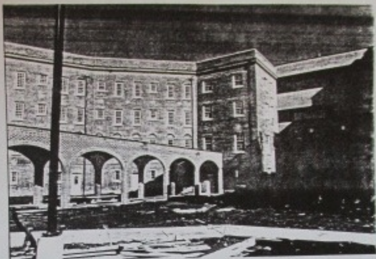
REAR VIEW OF EAST WING OF OLD BUILDING AND CONNECTION TO NEW BUILDING
